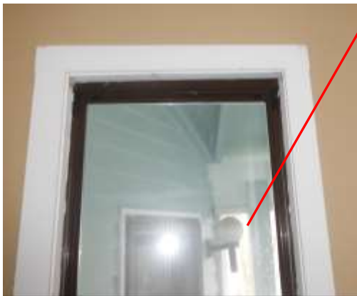
Figure 6 Window gaps, canted frames, and improper installation.
