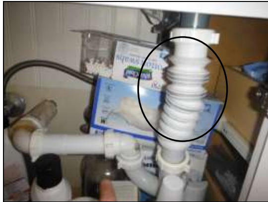
Figure 10 Unconventional/handyman or improper drain installation. Water getting behind the tub faucet handles; corrosion & calcium build-up. Have a licensed plumber evaluate and make all plumbing repairs.
