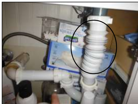
Figure 2 Unconventional/handyman or improper drain installation. Water getting behind the tub faucet handles; corrosion & calcium build-up. Have a licensed plumber evaluate and make all plumbing repairs.
