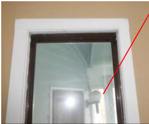
Figure 14 Window gaps, canted frames, and improper installation.
